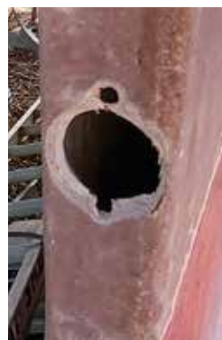
GRP around the stern tube's lower bolt hole was compressed to such an extent that it failed
