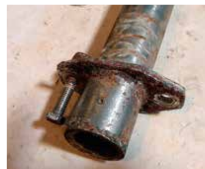
Stern tube withdrawn from the keel. A failed bolt hole in the keel GRP had allowed it to wobble
